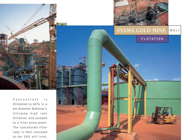
thickened to 60% in a 6m diameter Bateman's Ultrasep high rate thickener and pumped to a filter press plant. The concentrate filter cake is then conveyed to the SAG mill inlet, where the fuel content (as sulphide and organic carbon) supplements fuel addition to the existing whole ore roaster. This process considerably reduces fuel costs. Tailings are thickened similarly prior to being pumped to the slimes dam. Water recovered from the thickeners is recycled to a 1500 m³ mill return water tank.
