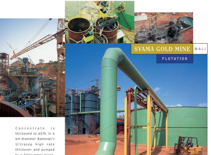
to a filter press plant. The concentrate filter cake is then conveyed to the SAG mill inlet, where the fuel content (as sulphide and organic carbon) supplements fuel addition to the existing whole ore roaster. This process considerably reduces fuel costs. Tailings are thickened similarly prior to being pumped to the slimes dam. Water recovered from the thickeners is recycled to a 1500 m<sup>3</sup> mill return water tank.
